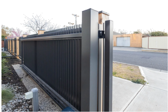
Black powdercoated fence and sliding front gate 1.2 m high
